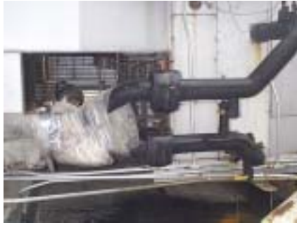
Examples of loss of energy due to poor insulation on HVAC systems
