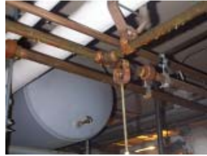
Examples of loss of energy due to poor insulation on HVAC systems
