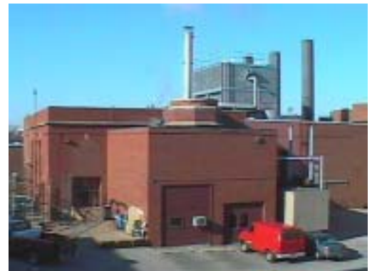
Illinois State University Power Plant
