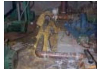
Poor Insulation in Mechanical Rooms
